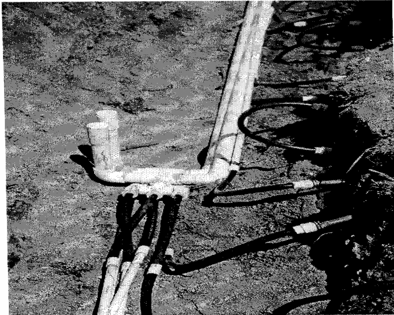
Figure 4-17. Pressure manifold and flexible drip lines prior to trench filling
