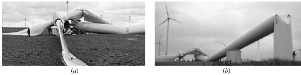
Figure 12. Examples of catastrophic collapse of wind turbines.
