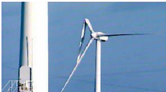
Figure 14. An example of blade damage near 30% in length from the blade root.
