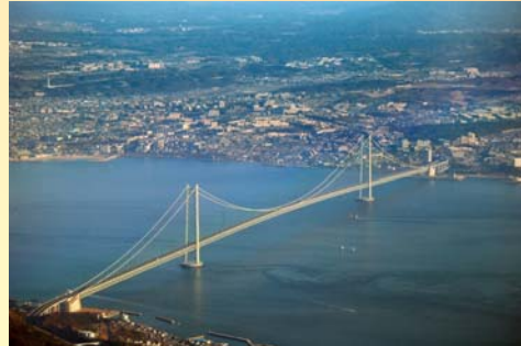
Akashi Kaikyo Bridge 6532 ft.
