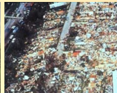
1992, Hurricane Damage, Miami
