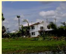
2004, Hurricane Damage, Tampa
