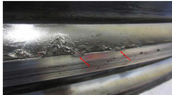
Bearing Damage from Ellipse Spill
