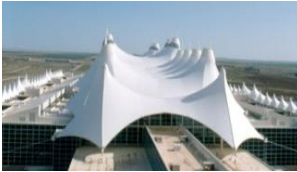
Tension Fabric Denver Airport
