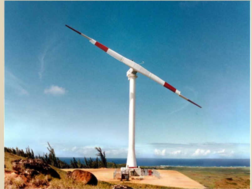
MOD-5B Wind Turbine (Two-bladed, teetered hub, 3.2 MW)
