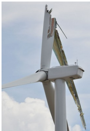
Failure of a 49 meter wind turbine blade wind-watch
