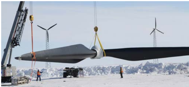
Blade installation in Kotzebue Alaska, used with permission KEA
