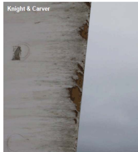
Blade: erosion on the leading edge
