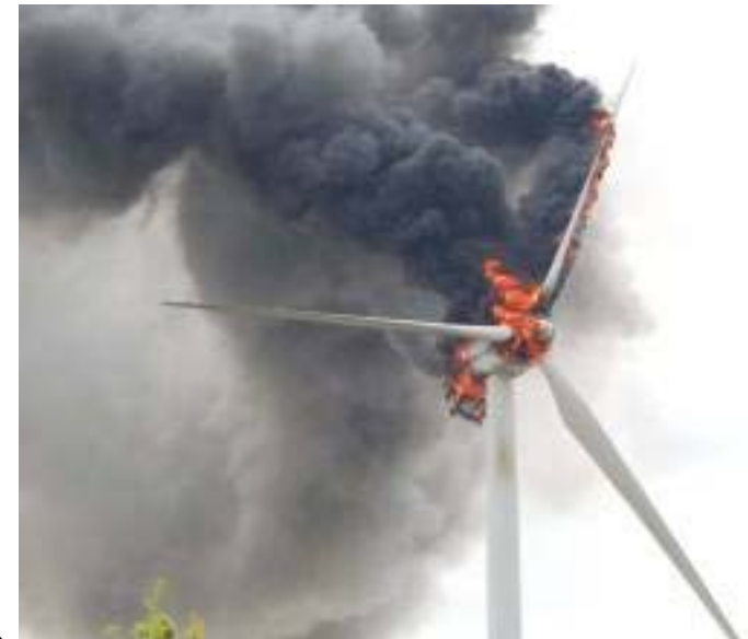
Blade damage: lightning strike
