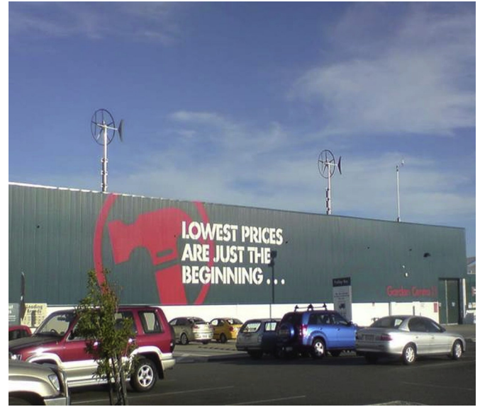
Fig. 3. Position of the ultrasonic anemometer on the roof of the Bunnings warehouse in Port-Kennedy, Western Australia.
