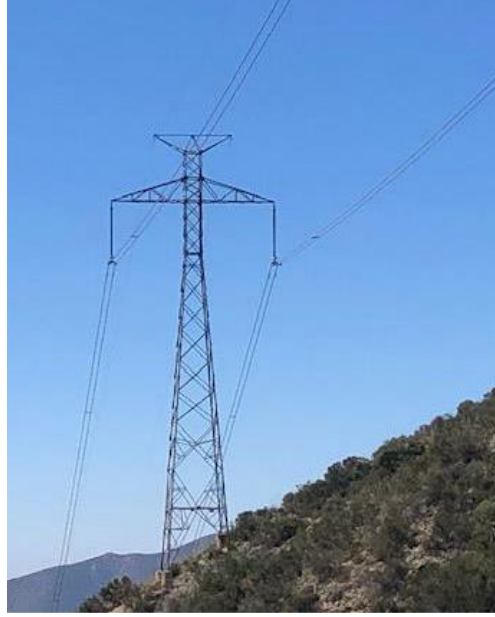
Figure 7a - 17: A tower for the PDCI showing two conductors per pole
