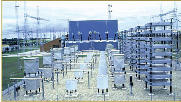
**figure 1.** HVDC converter station with ac filters in the foreground and valve hall in the background.
