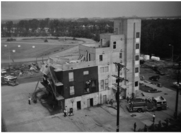
Figure 9: The Burn Building in Rockville, MD: site of the DARPA TMR Demo.
