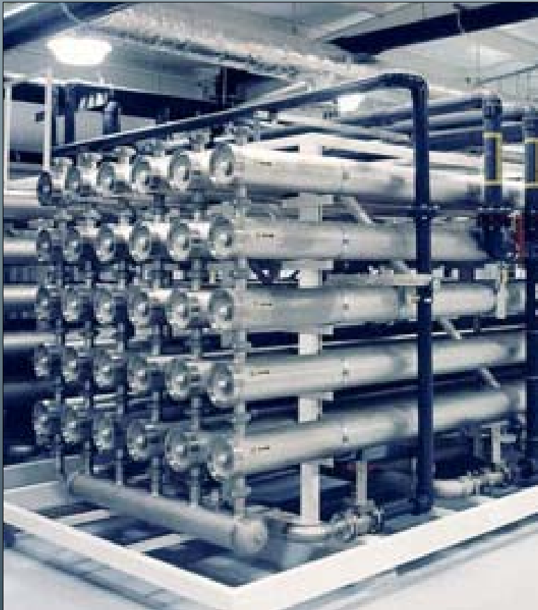
Figure 6: Typical RO desalination plant
