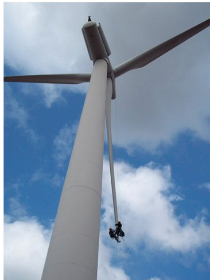
Technicians must inspect, clean and repair the composite rotor blades whose good condition is vital to wind turbine efficiency. (Pictures courtesy of BS Rotor Technic (UK) Ltd.)
