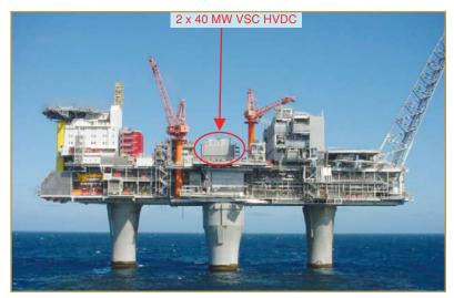
figure 11. VSC power supply to Troll A production platform.
