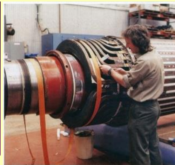
Repairs to the overhand insulation of this 200MW generator rotor were carried out by experienced tradesmen working on shift to ensure the earliest possible return to service.
