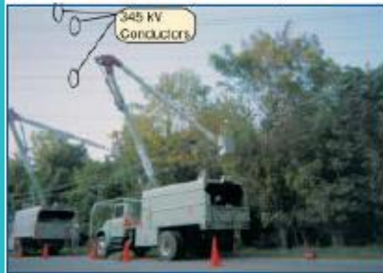
This August 14 photo shows the tree that caused the loss of the Hanna-Juniper line (tallest tree in photo). Other 345-kV conductors and shield wires can be seen in the background. Photo by Nelson Tree.
