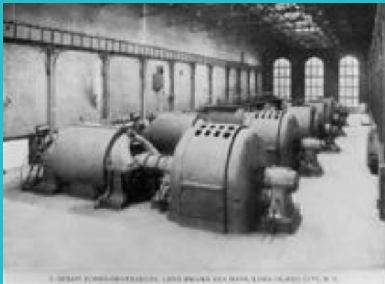
Steam turbo-generators, Long Island railways, c.1907
