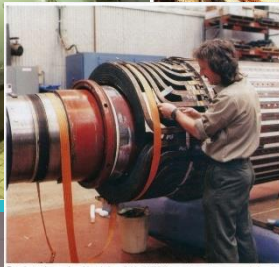
Repairs to the overhead insulation of this 200MW generator rotor were carried out by experienced tradesmen working on shift to ensure the earliest possible return to service.
