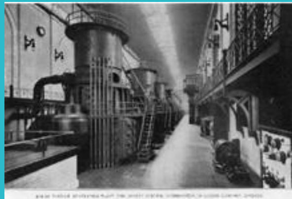
Fiske Street Station steam turbine Chicago, c.1907
